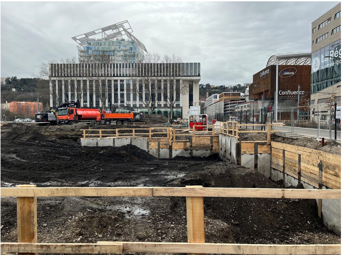
Construction of Zephyr foundations (February 2026)
